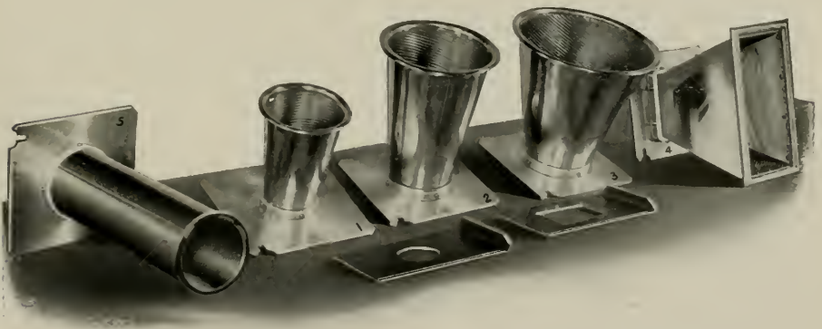
Fig. 327. A and AA, lead which protects the plate against the action of the X-ray. B, window of thin aluminum or celluloid on which the part being radiographed lies. C, end of the tunnel. D, plate carrier. E, end of 5x7 plate on which the first radiograph is made with the tube in position I. EE, end of plate on which second radiograph is made after it is shifted under the window B, and the tube is in position J. F, centering line. G, angle of X-rays with the tube in the first position, I. H, angle of X-rays with the tube in second position, J. The diagram shows the tube being shifted on a line with its long axis. It may be shifted in this manner, or at any angle to its long axis—it makes no difference.
